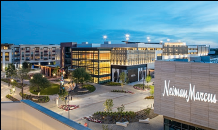
▲ THE SHOPS AT CLEARFORK Ft. Worth, TX
